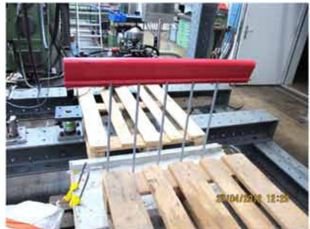
d) Arrangement of reinforcing bars, \varnothing 14 mm for V01-14, n=5 , a=150 mm, L=650 mm
