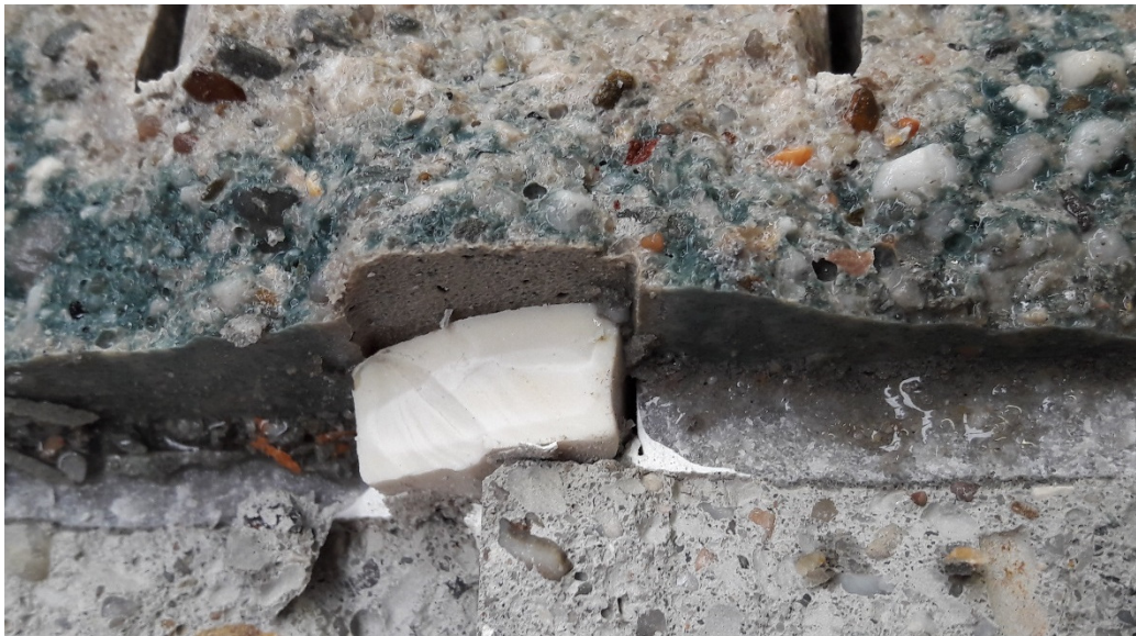
Photo 3. Configuration C, Detail of PC Elastoswell, no leakage visible
